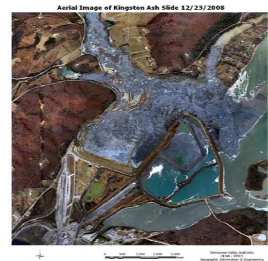
TVA Kingston Power Station after the December 2008 coal ash spill.
